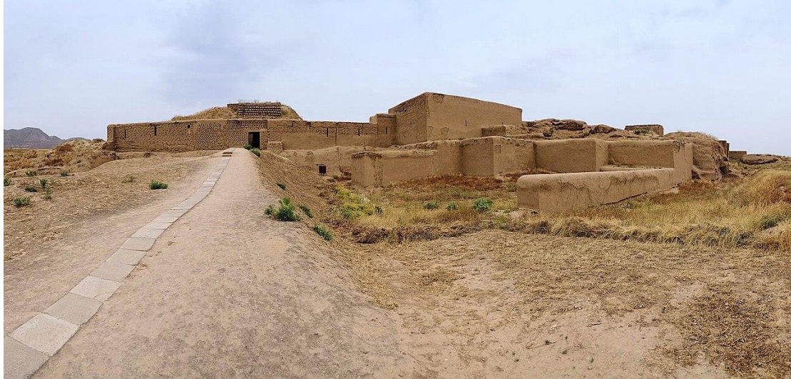
Mithradat-kert (literally the city of Mithridates I of Parthia) in today's Nisa (or Nissa or Nusay) in Eastern Turkmenistan; the entrance to the city and the walls, which had to be covered up to prevent further damage from erosion
